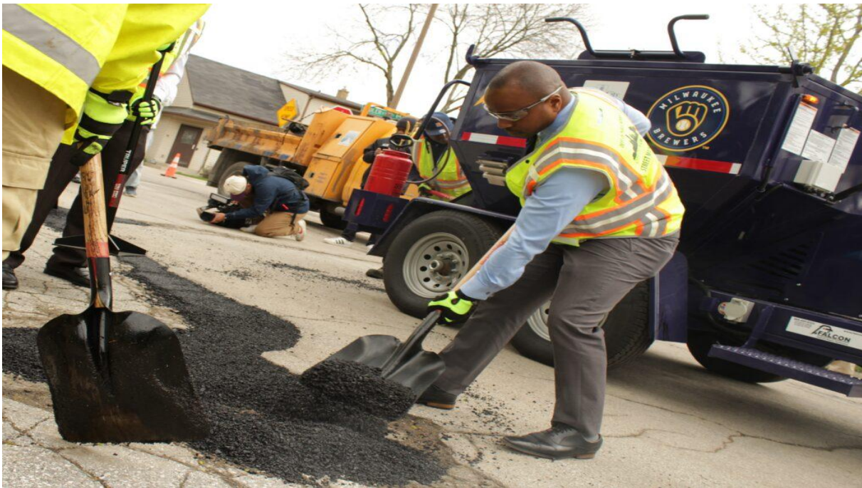
Milwaukee DPW / Brewers pothole-repair partnership with Mayor Cavalier Johnson filling holes at the rollout of the DPW hot box trailer purchased by the Brewers. This item ties to auto centric and external partnerships categories outlined in the report.
